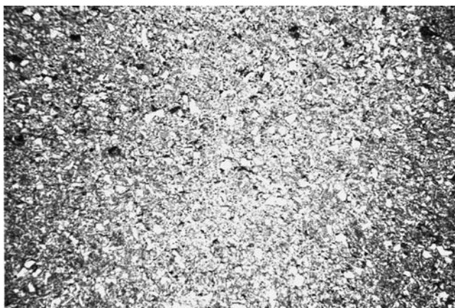
Figure 10. Popouts and raveling in 2-year-old pavement.
