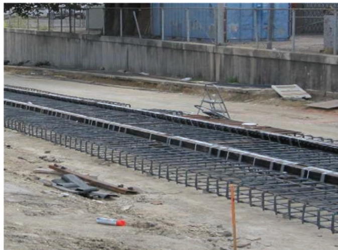
Figure 16. Steel reinforcement for the embedded slab track.
