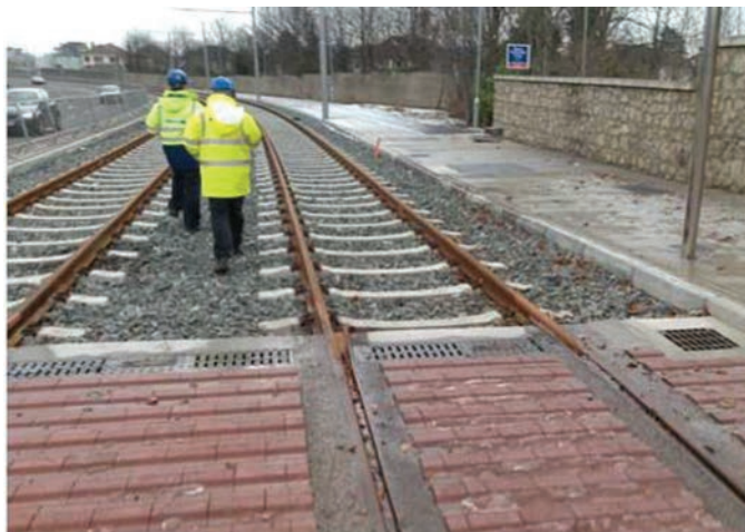
Figure 22. Embedded and ballasted section.
