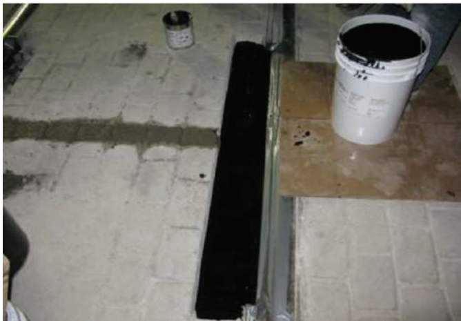
Figure 23. Iso-flex replacing rail boot.
