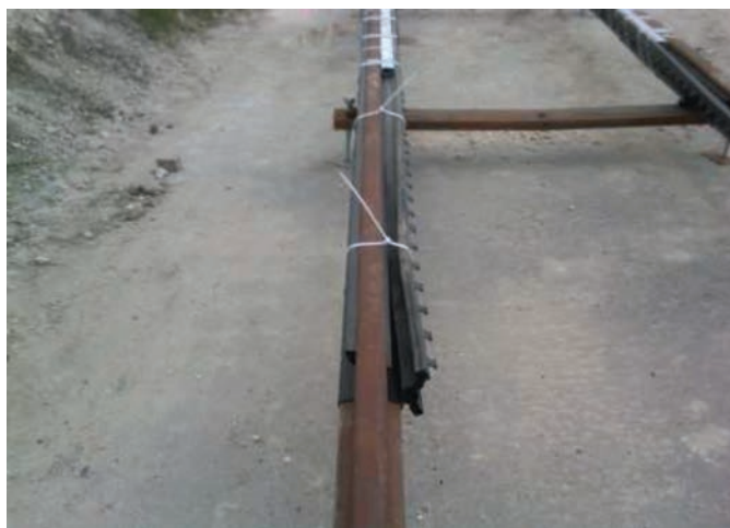
Figure 15. Section of flangeway filler rail boot during construction.
