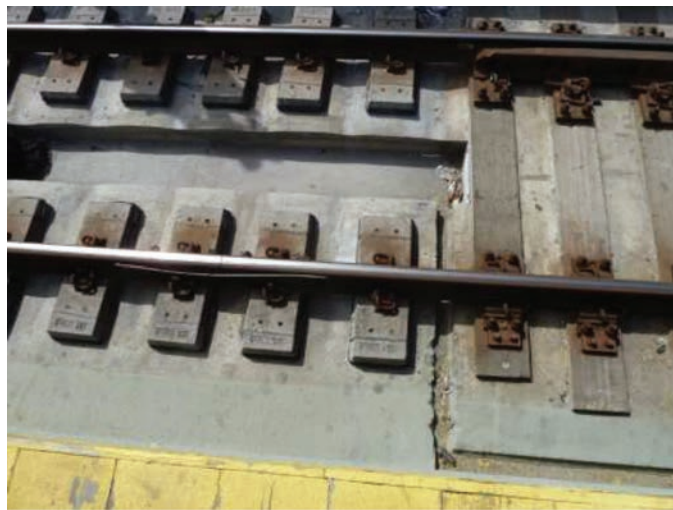
Figure 19. Section of ongoing construction with concrete and wooden ties.
