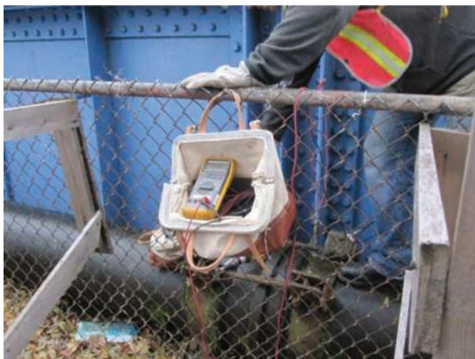
Figure 20. Water pipe utility test on bridge.
