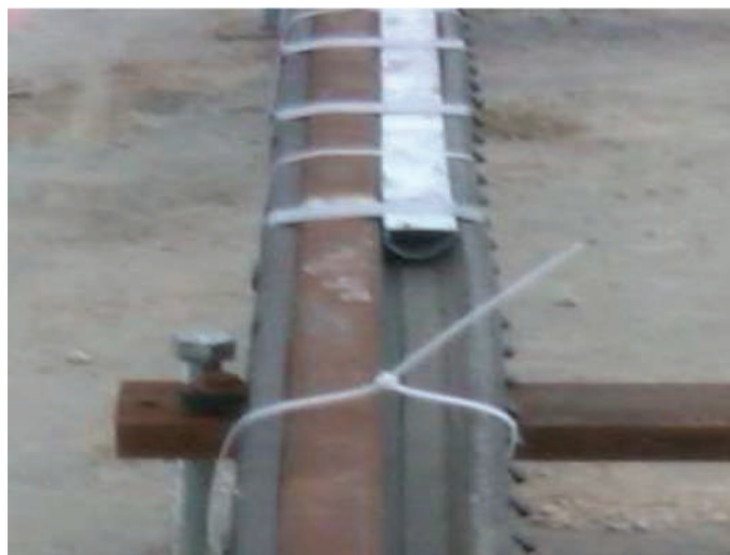
Figure 13. Tee rail with grooved rail boot.
